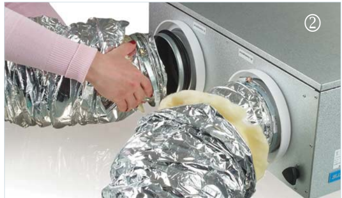
Cover the air handling unit spigots with the inner hoses of the heat-insulated air ducts and fix those with metal clamps (special accessory).
