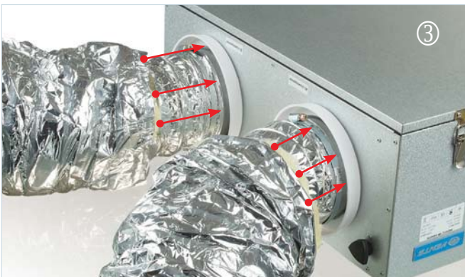
Tuck the inner insulation layer of the air ducts under the flanges of NM Isovent mounting kit.
