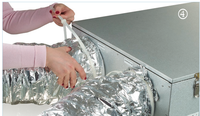
Cover the flanges of NM Isovent mounting kit with inner hoses of heat-insulated air ducts by pressing the hoses tightly against the air handling unit casing and fixing those with clamps (included into delivery).
